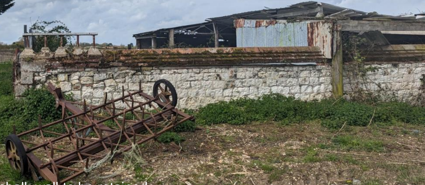
East boundary, chalk wall to be retained
